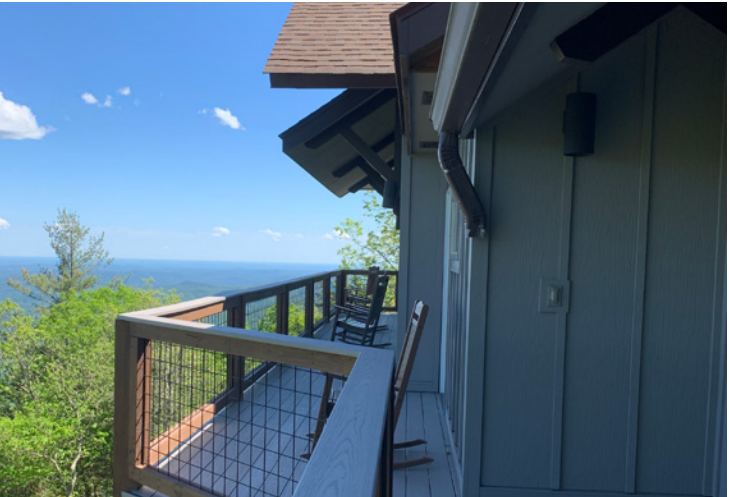
Lodge siding replacement on the east and north sides, a much-needed project to protect the integrity of this building.
