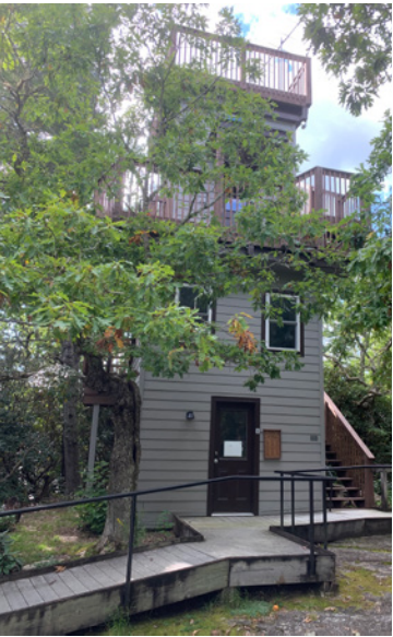
The tower renovations included upgrading the structure, providing a new meeting space, office, and a new roof.
