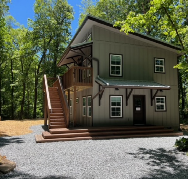
Since 1979, improved staff housing has been a major goal. Weve come a long way from the trailer demolition to beautiful new housing and it means so much that this has become a reality.
