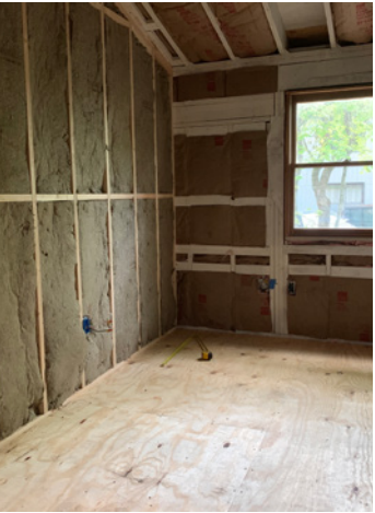
Beginning renovation on cabins 9 and 10
