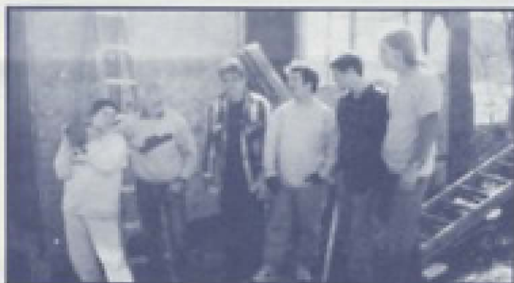
Mountain Staff and REFUEL renovating Cabin 12
