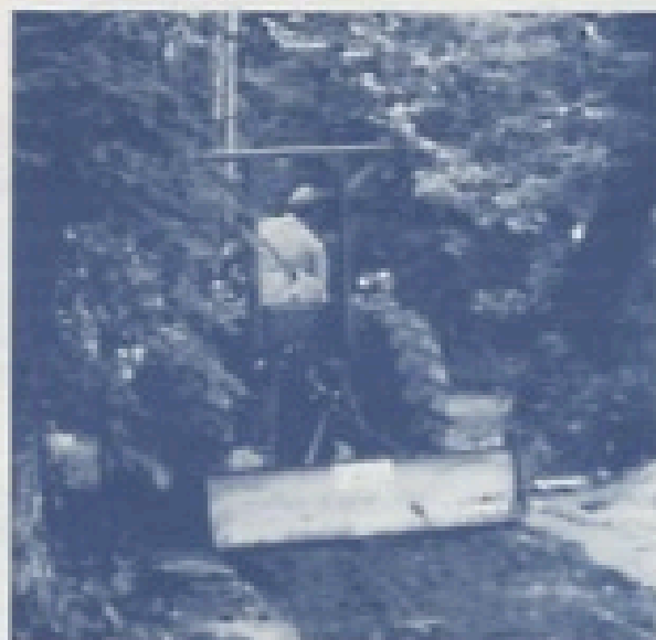
Preparing the new pathway from the Lodge to Cabin 1.
